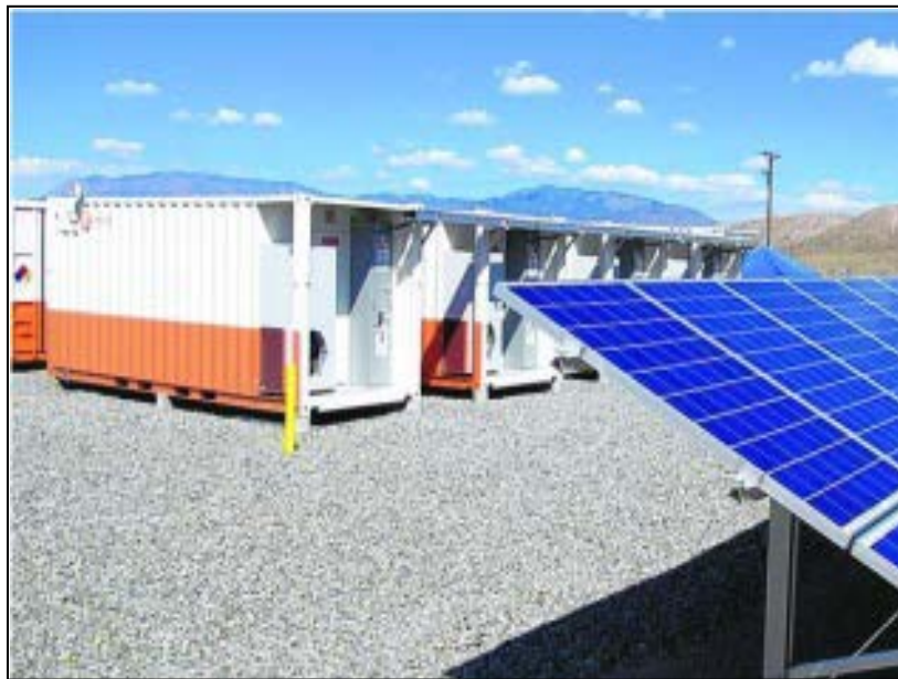
Figure 73. 500-kW/1-MWh Advanced Lead-acid Battery for Time-shifting and 900-kWh Advanced Carbon Valve-regulated Battery for Photovoltaic Smoothing This is a solar energy storage facility that is fully integrated into a utility's power grid. (Source: PNM Resources)
