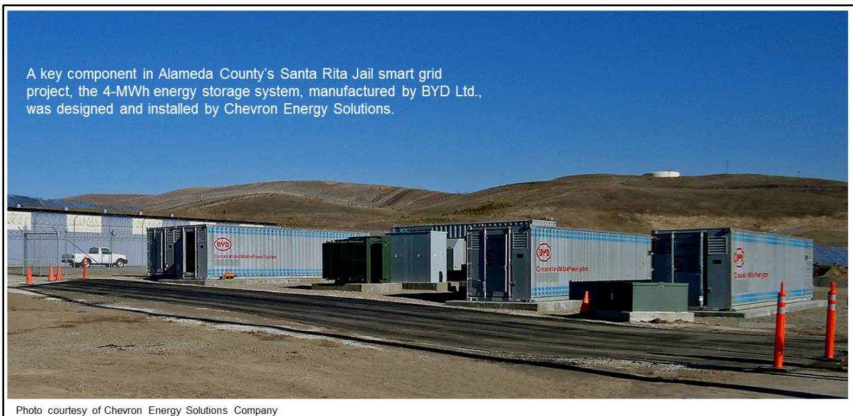
Figure 98. A 2-MW/4-MWh Li-ion Energy Storage System
